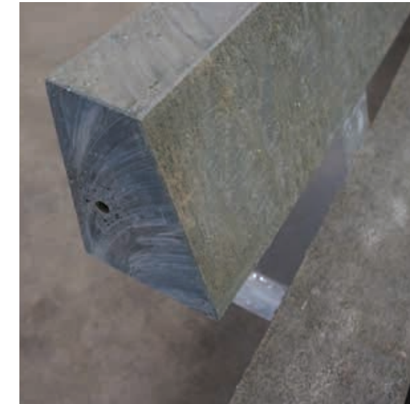
Detail Luft einschlüsse
