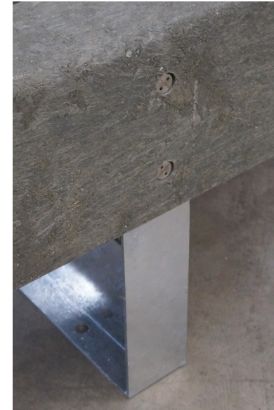
Detail Streetlock® Anti-diefstal moeren
